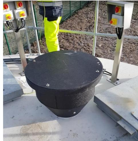
Figure 1 - Anua Clean Air ACU-600 - Passive Activated Carbon Unit
