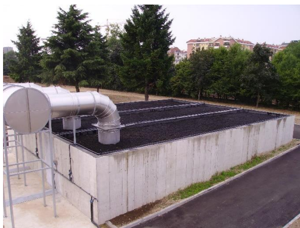
Figure 1 - Mónafil Installation in Milan, Italy
